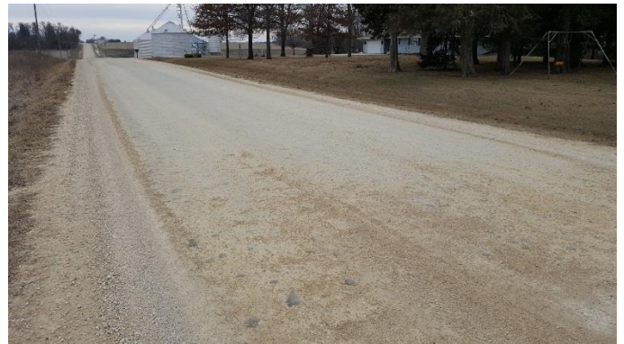
Calcium chloride was applied to the crushed stone road approximately 7 months prior to the picture for dust suppression.
